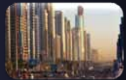
Building Security Control
